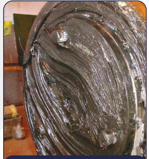
Slow speed bearing from an oven motor, after being removed for replacement
